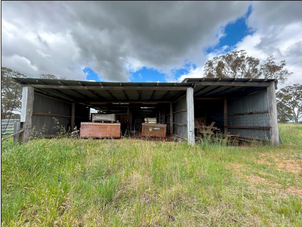
Site Photograph 5.3 View of sheet metal storage shed, identified in the western portion of 241 Grafton Road, as observed facing south on 15 October 2024 by SE (2024). Consistent with observations made during the investigation conducted on 3 March 2026.
