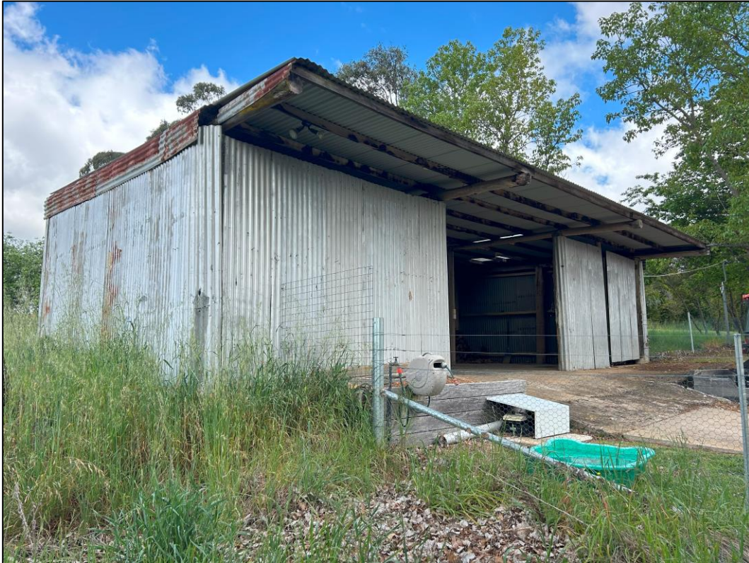
Site Photograph 5.2 View of sheet metal shed, located adjacent to the residence in the south-western portion of 241 Grafton Road, as observed facing south-west on 15 October 2024 by SE (2024). Consistent with observations made during the investigation conducted on 3 March 2026.
