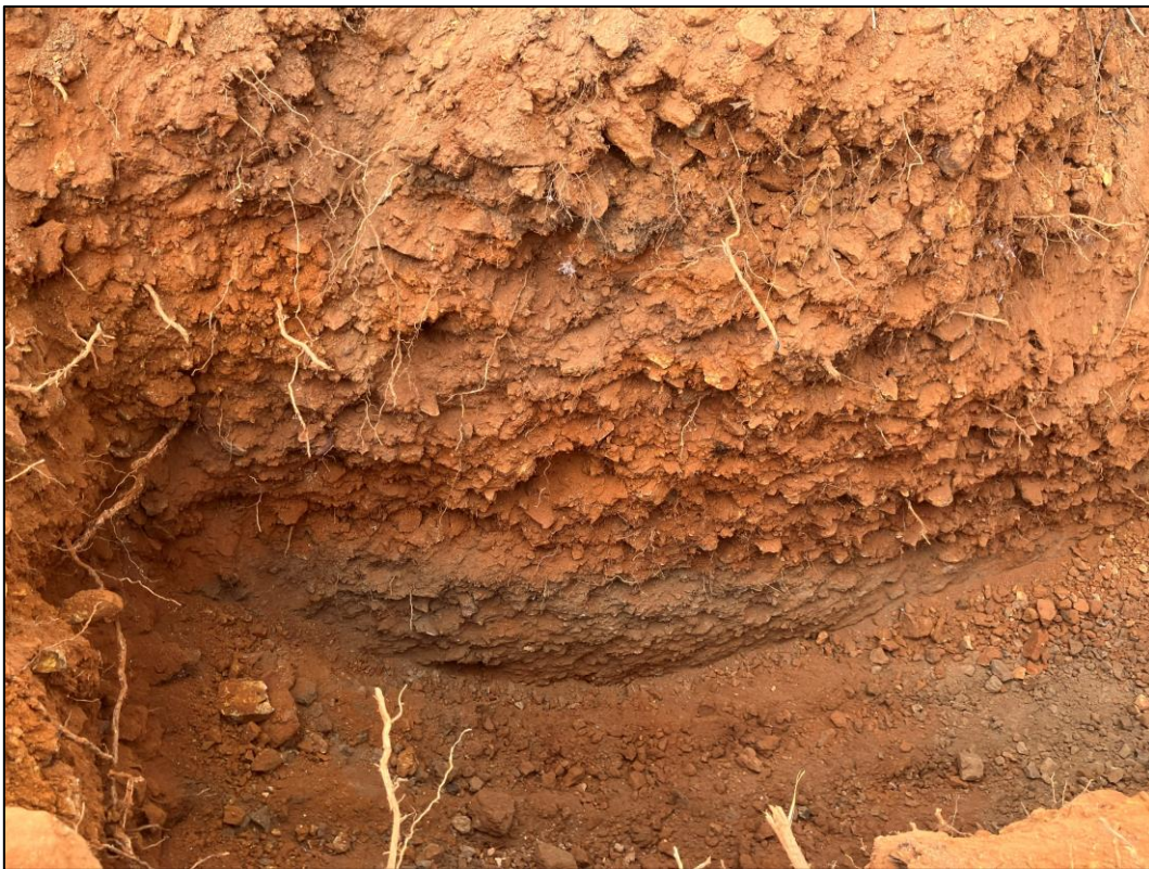
Site Photograph 13.1.3 View of CLAY fill material identified within the former dam located south of the main residence, as observed 3 March 2026.
